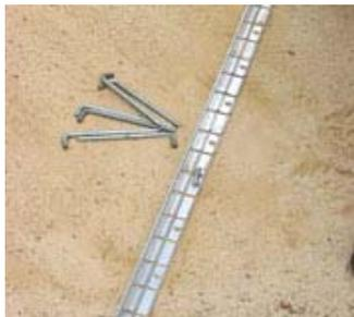
8. Once satisfied with the positioning of the LINKedge, hammer spikes firmly into the ground using a hammer.
