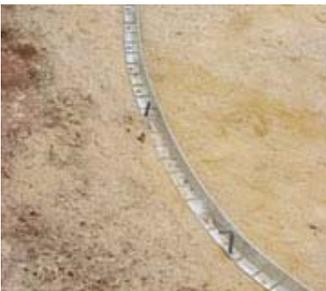
4. Half hammer subsequent spikes in pivotal areas along the length. (especially at points where a bend or curve are required)
