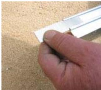
5. Connect any further 3m lengths together by using the provided fishplate. Slide the fishplate into the designated section at the end of the length.
