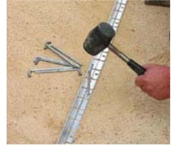
3. Half hammer spikes into pre punched holes (approx 4 spikes every 3m length) starting from the first hole in the end of the LINKedge
