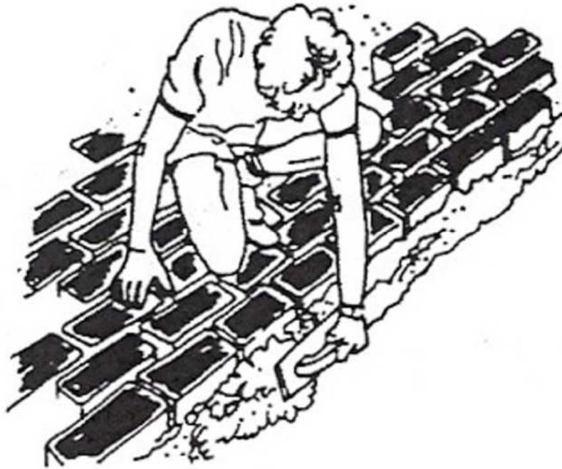
Edge restraints are necessary to retain and restrain the paving units and sand. Otherwise, paving failure may occur.
